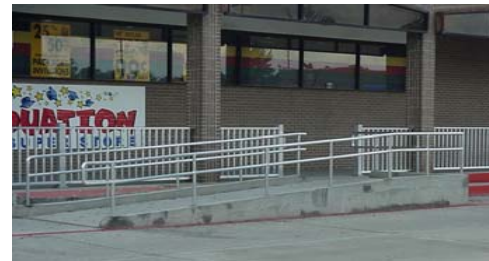
Handrail with handicap access rail
